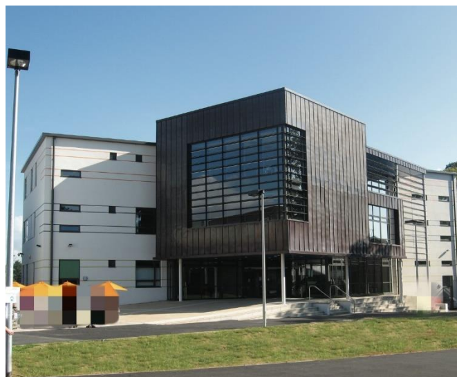
Figure 2. The building studied.
