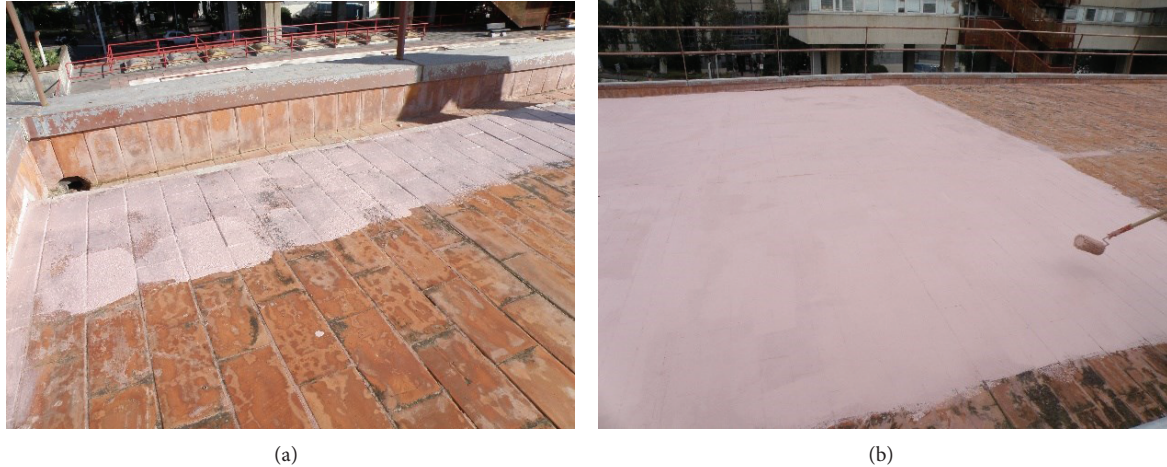
FIGURE 4: Application of the cool paint on the existing clay tiles.
