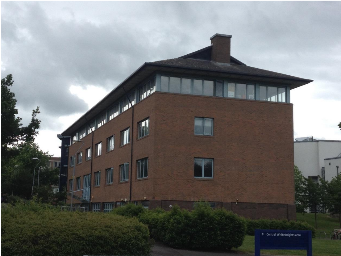
Figure 2.3 the HBS building
