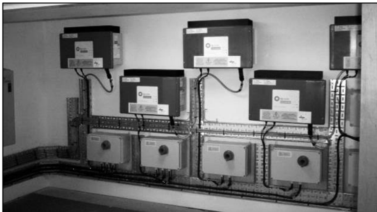
Figure 2-8: Inverters and isolators
