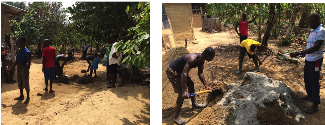
Photo 4.5: Communal labour constructing clinic in Kamaso Source: Author (2016)
