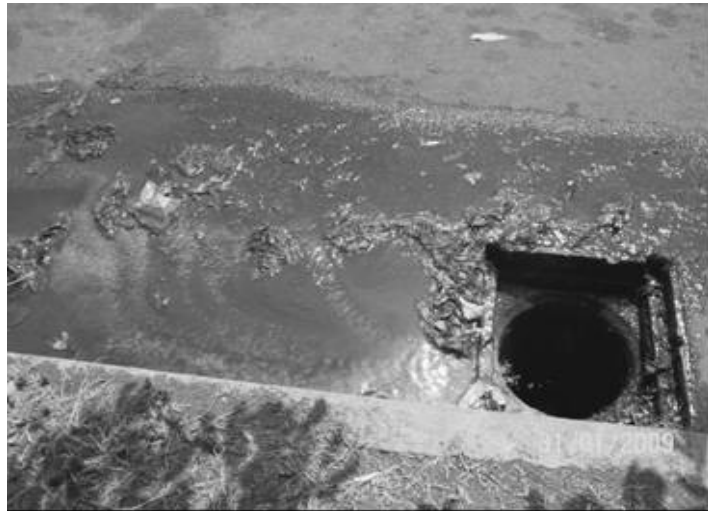
Plate 2: Sanitary system overflow at Garki District
