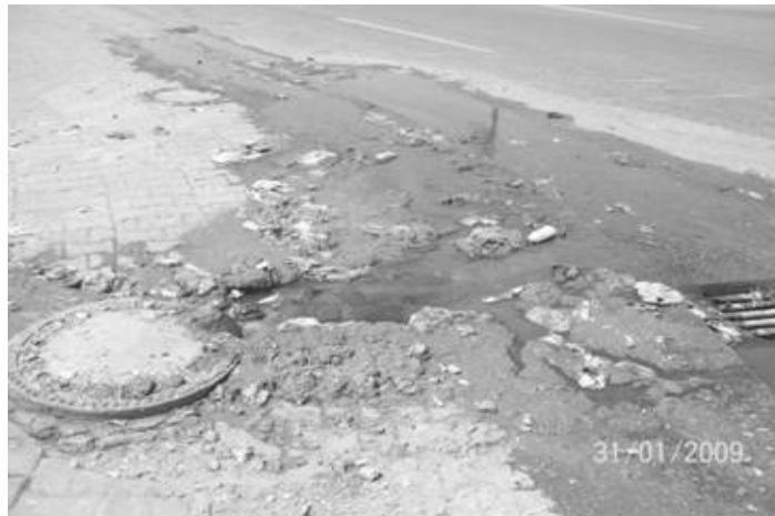
Plate 1: Sanitary System Overflows at Wuse District
