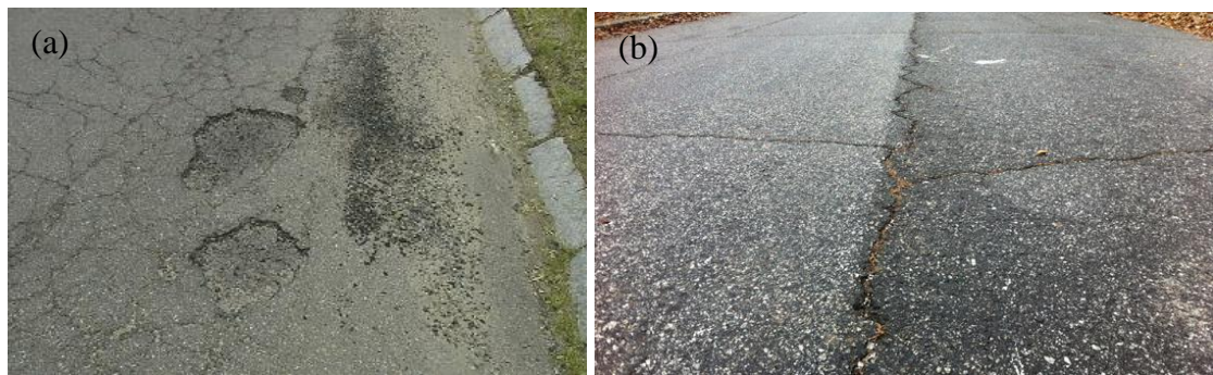
Figure 1. 3 Photographs of examples of (a) fretting and (b) transverse and longitudinal cracking within a road surface
