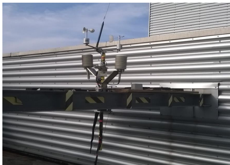
Figure 1. 19 Photograph of the weather station on the roof of Crowthorne House
