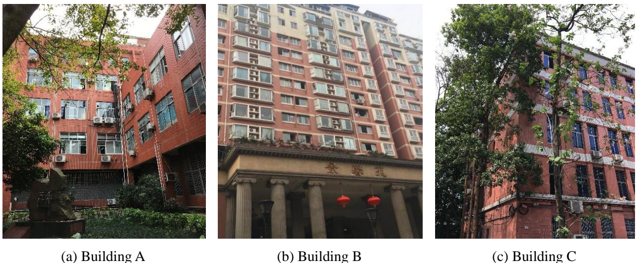
Fig.2. Three office buildings considered in this study
