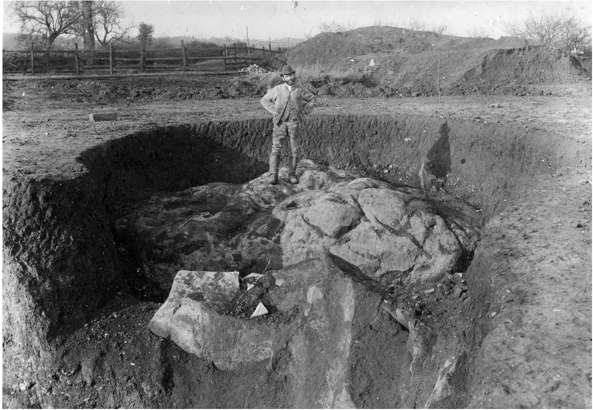
Figure 4 Sarsen quarrying at Denner Hill, Buckinghamshire, c.1907 (© Buckinghamshire County Council, HG33).
