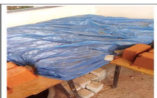
Figure 4 CSEBs covered with blue plastic sheet during curing
