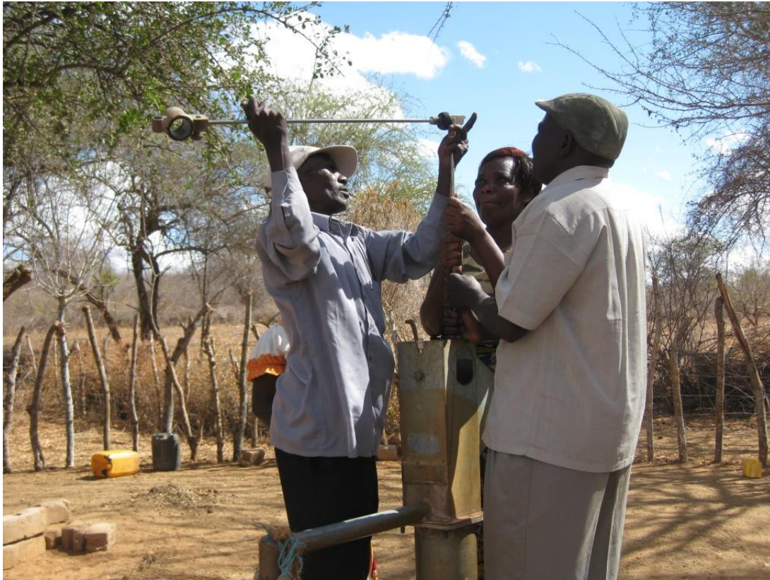
Picture 1: Rufus Mwaniki of repairing a handpump (credit: Tim Foster)
