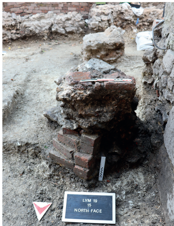
Fig 28. North face of north foundation pier (15) showing recent brick underpinning. Photograph: authors.
