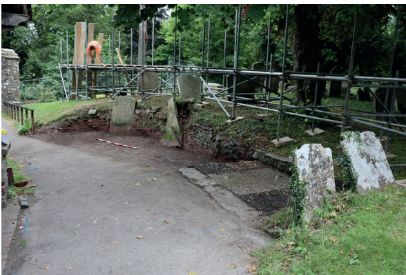
Fig 11. View in front of south porch before 2019 excavation showing mid-twentieth tarmac path and nineteenth-century niche (with headstones) constructed to display the foundations of the Anglo-Saxon apse. Photograph: authors.
