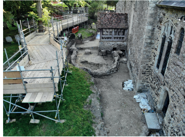
Fig 12. View of church foundations viewed from the east; the north wall of the nave can be seen running under the south porch. Photograph: authors.
