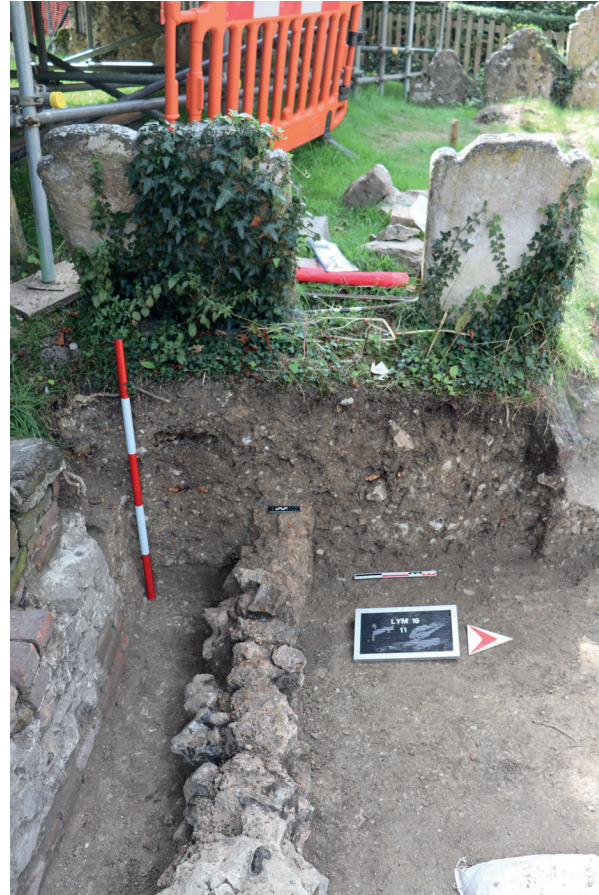
Fig 34. Foundation of south nave wall. Photograph: authors.
