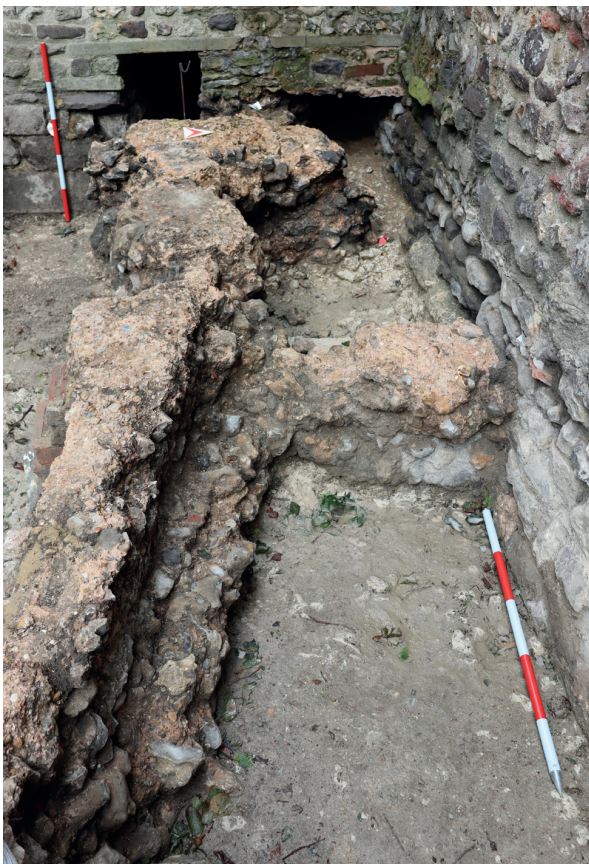
Fig 26. Fragment of wall projecting from the north side of the apse truncated by the south wall of the nave of the extant church. Photograph: authors.
