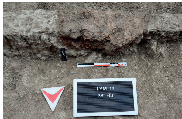
Fig 35. Sliver of in situ foundation (36) for the west wall. Photograph: authors.
