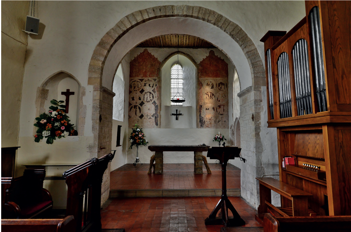
Fig 42. St Mary, Brook, Kent. Chancel arch of c 1096–1107. The Early English east window is probably a modified Norman opening. Image: © Michael Garlicke, https://creativecommons.org/licenses/by-sa/2.0/
