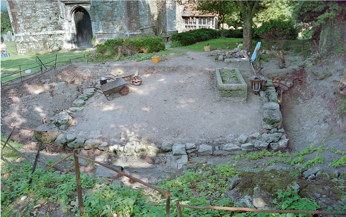
Fig 39. View of 1991–3 interventions in progress. Photograph: authors.
