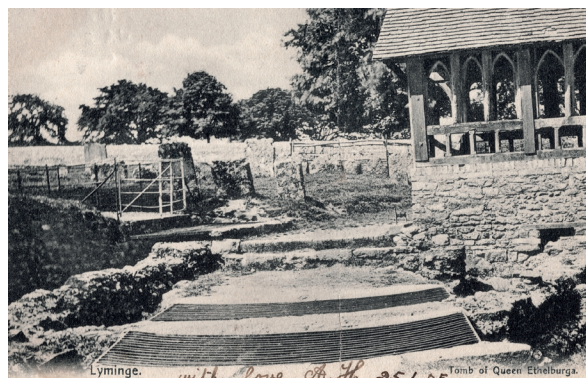
Fig 17. Postcard post-dated 25 Jan 1905 showing exposed foundations with surmounting path with iron display grills. Image: from the collection of and © Robert Baldwin.
