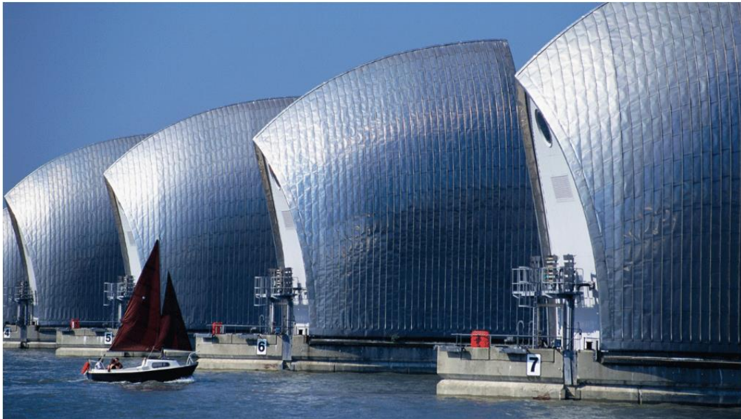
FIGURE 3.4. THE THAMES BARRIER. SOURCE: COSTAIN 2015
