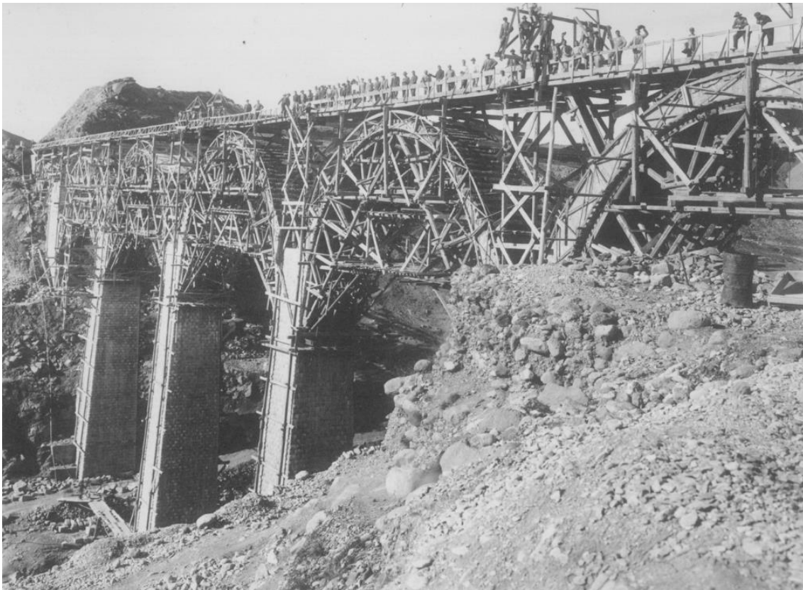
FIGURE 3.3. CONSTRUCTION OF THE TRANS-IRANIAN RAILWAY. SOURCE: COSTAIN 2015
