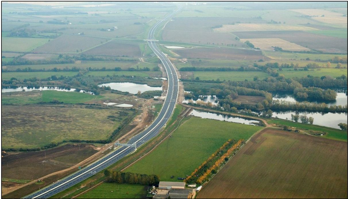
FIGURE 3.11. PHOTOGRAPH OF THE A14. SOURCE: COSTAIN 2019
