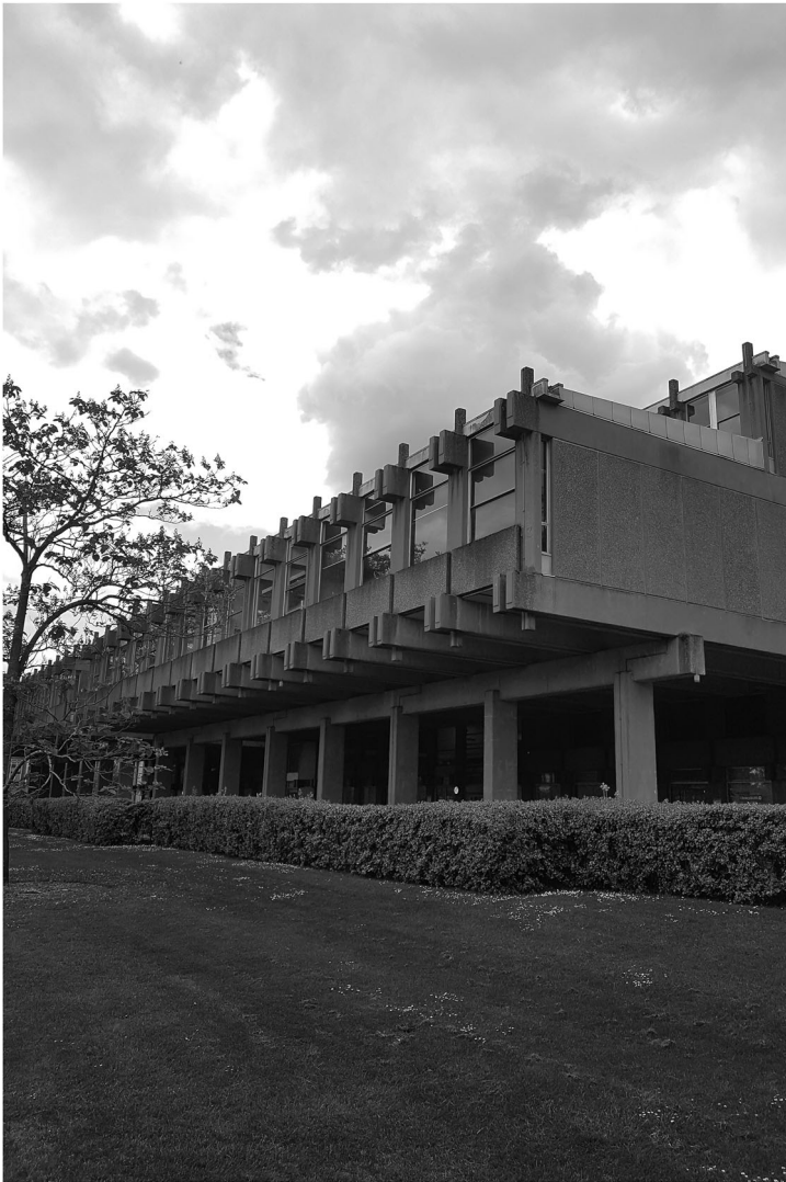
Figure 1. The external envelope of the URS building.
