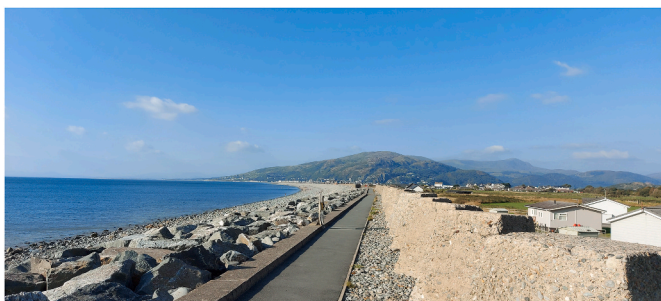
Fig. 1. Fairbourne's shingle bank and reinforced crest wall.
