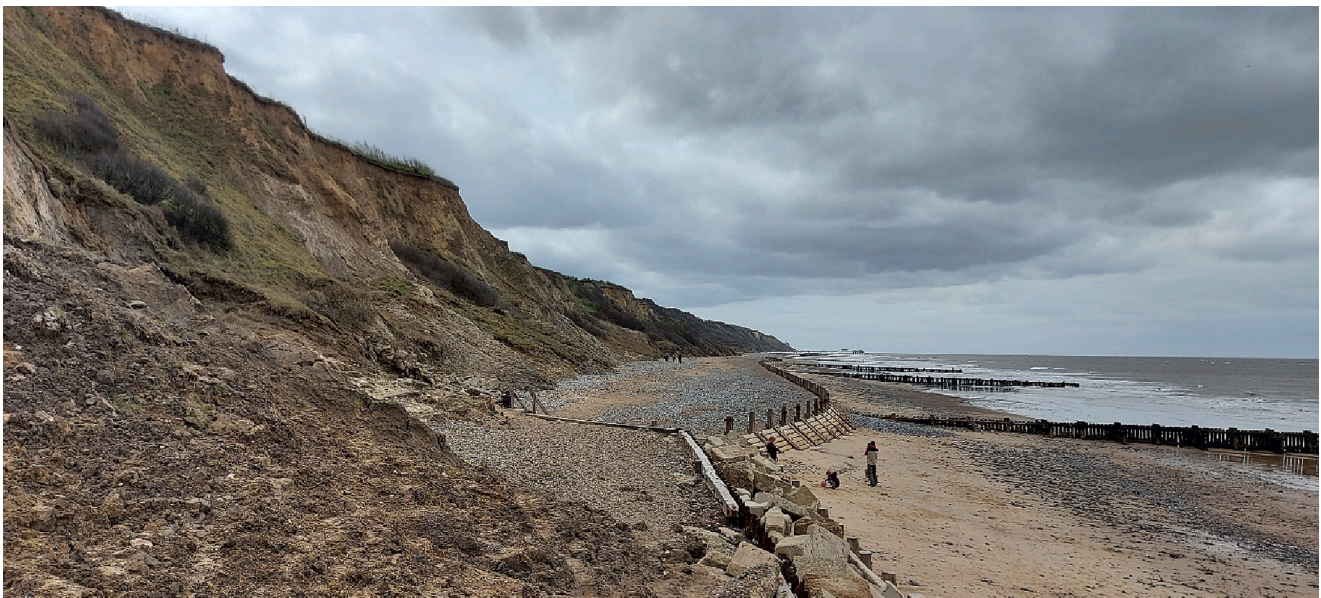
Fig. 4. View of Overstrand beach, looking northwest towards Cromer. Groynes and revetments are visible on the beach. On the left, the presence of fresh earth indicates recent slumping of the marine cliff (credit: author's photograph).
