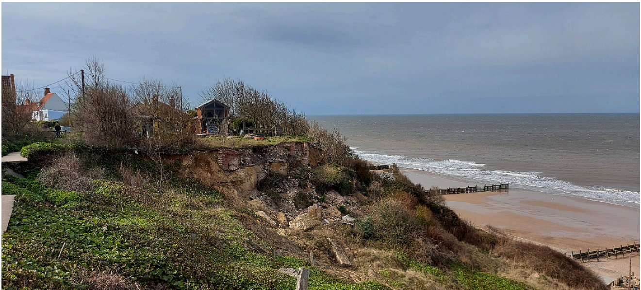
Fig. 3. Coastal buildings collapsing down the cliff face, Overstrand, UK. Wooden groynes are visible on the beach (credit: author's photograph).
