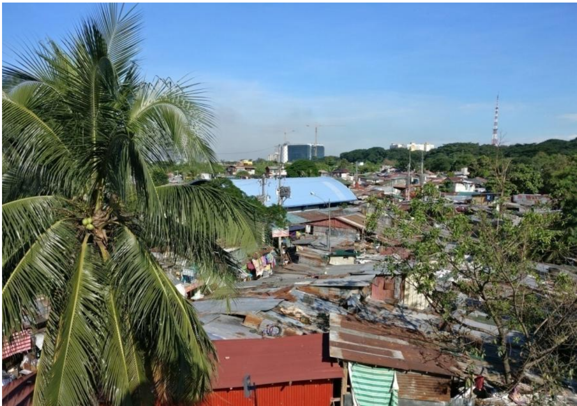
Figure 21 Distinctive Roof Profile of the Covered Court from the footbridge
