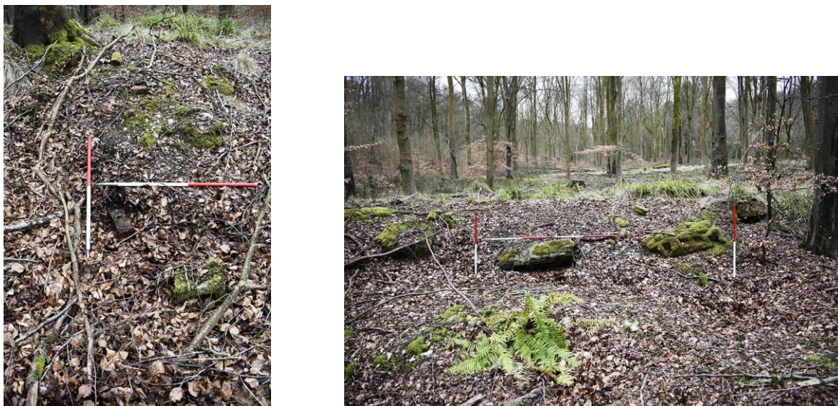
Figure 24 Left: bricks on the surface and eroding from the southern scarp of finger-dump [10]. Right: large concrete blocks on its northern scarp.
