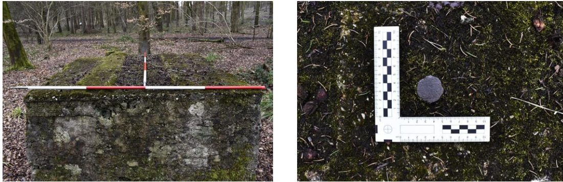
Figure 29 Left: the top of the concrete block. Right: one of the iron pins in the top of the concrete block.
