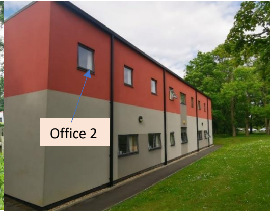
Figure 4.7: South facing elevation Building 2
