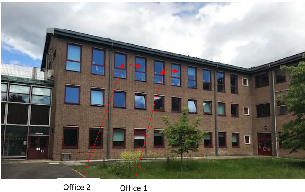
Figure 4.1: South facing elevation Building 1
