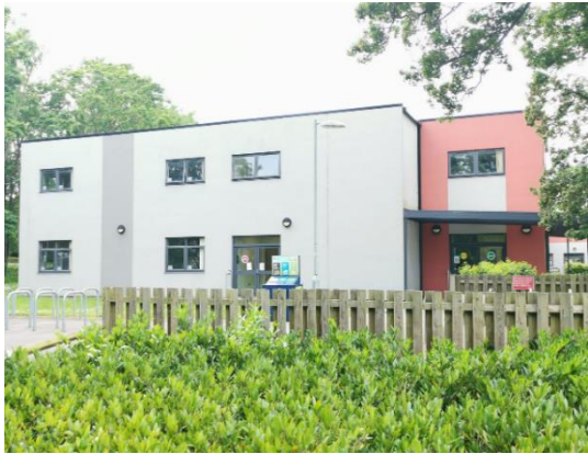
Figure 4.6: Front entrance and east facing elevation Building 2
