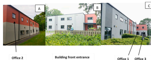
Fig. 1. Building elevations A = South facing B = East facing and C = North facing.
