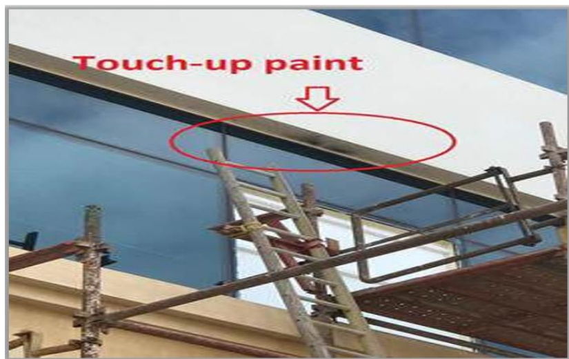
Figure 7.25 Touch-up Paint (Source: The maintenance team)
