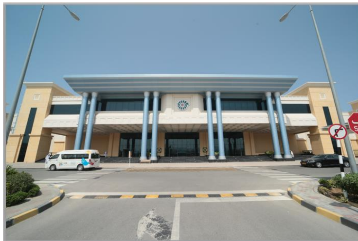
Figure 7.21 The Main Entrance (Source: Author)
