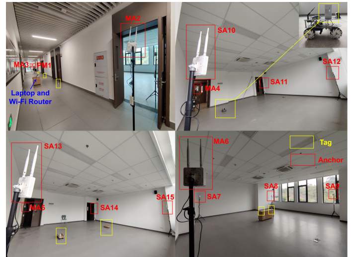
Fig. 15: Anchor deployment in the office space.
