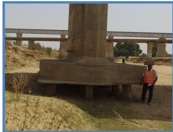
Figure 23. Exposed pile caps and piles
