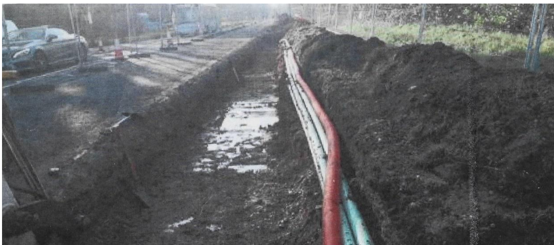
Figure 5. 4 Relocated fibre optic cables after widening the road on the (23/1/ 2020)
