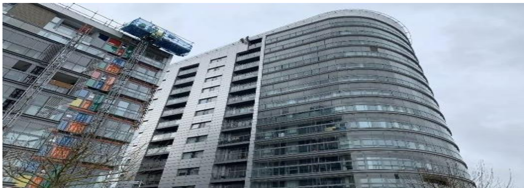
Figure 4. 5 New external cladding installed at block J
