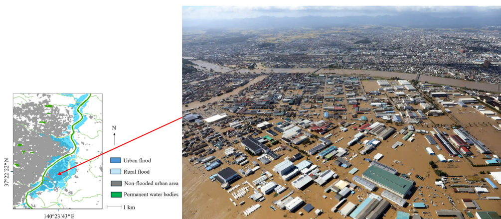
Fig. 3 Aerial photograph of the flooding viewed from the East. 43
