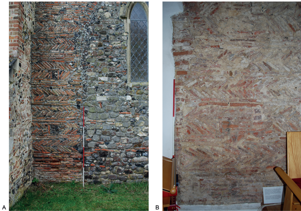
Figure 3. St John the Baptist, Reedham: (A) re-used Roman brick and tile at the east end of the nave on the north side; (B) internal elevation of (A): re-used Roman brick and tile at the east end of the north wall of the nave.
