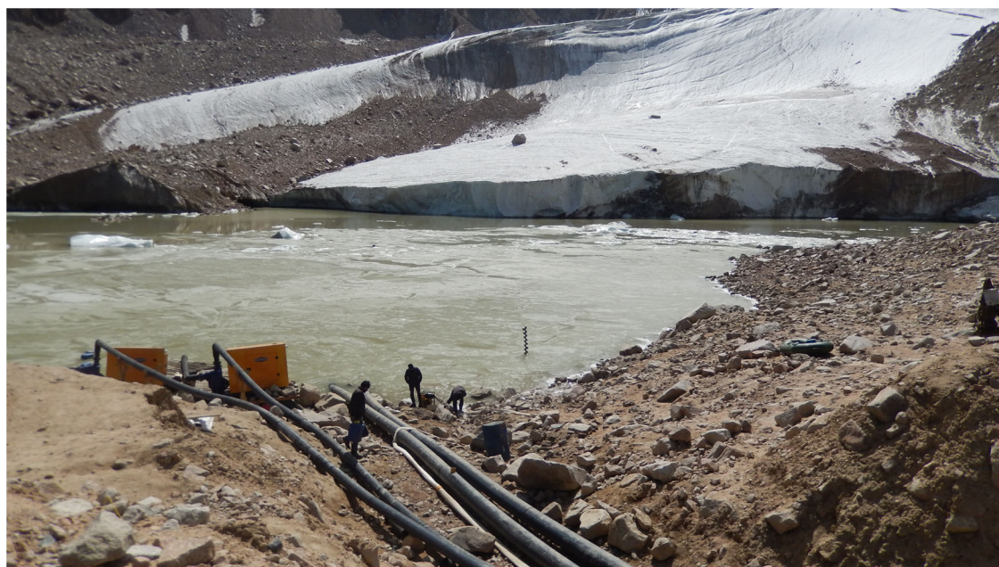
Fig. 8 | Preventive artificial drainage of Lake 13-bis in the UA catchment (43.039°N; 77.044°E). Photo: M. Shahgedanova.
