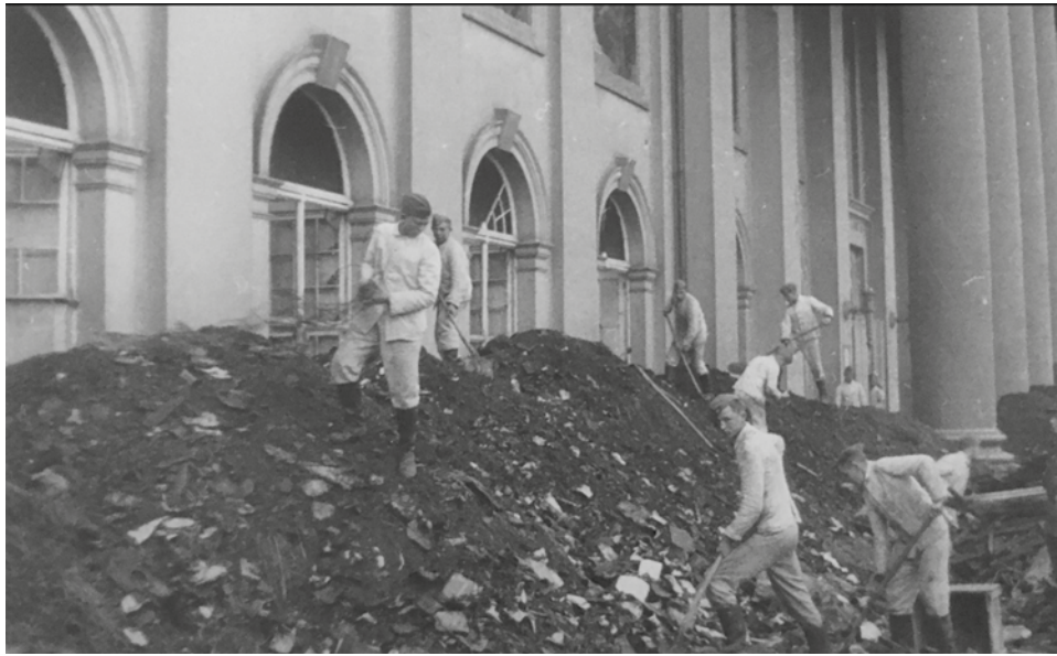
fig. 8. Clearing away war debris from Fridericianum after its bombing in 1943, Photographer unknown.
