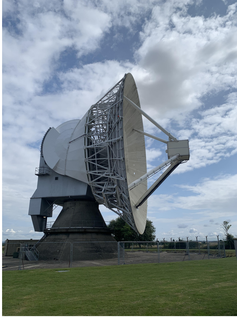
Figure 2.4: The 25 m antenna of the Chilbolton Advanced Meteorological Radar (CAMRa) located at the Chilbolton Observatory.
