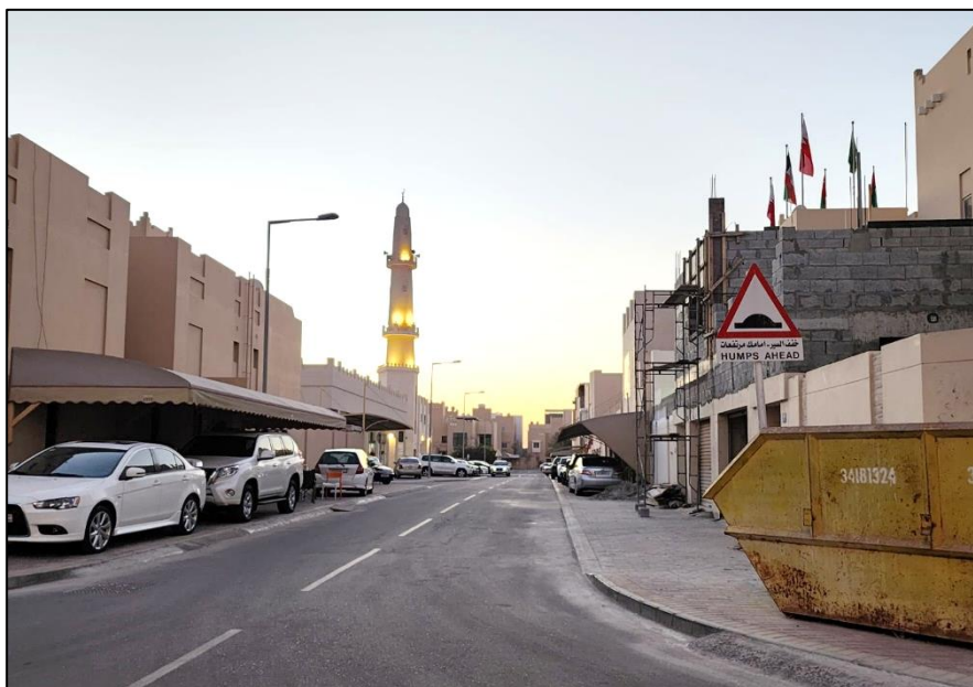
Figure 6.8. Unaltered original facades and absence of greenery in a section of the neighborhood, reflecting negatively perceived elements.
