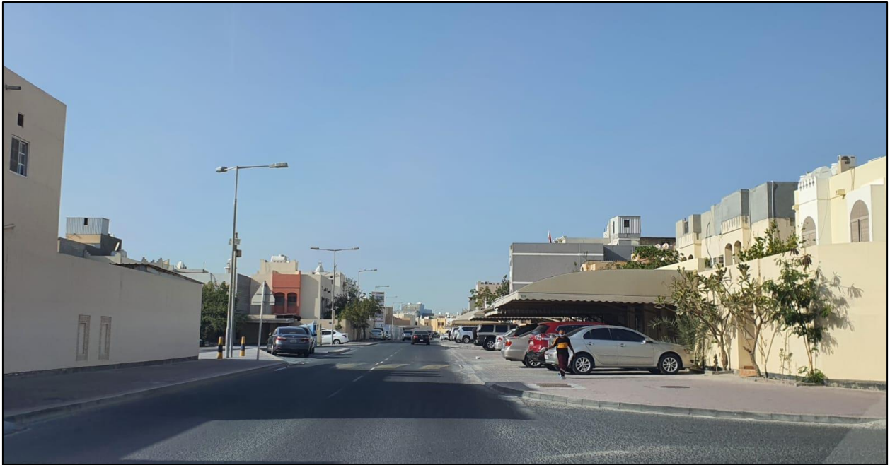
Figure 5. 17. A photograph taken for Alsayah Affordable housing neighbourhood
