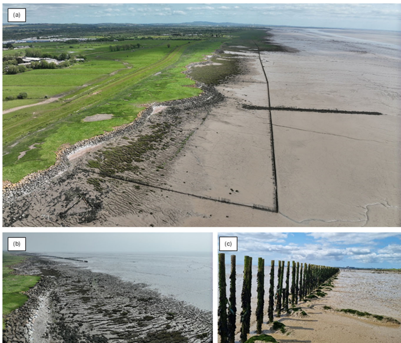
Figure 3. Imagery taken by the authors in May 2023 of (a) the western end (looking eastwards) of the Rumney Great Wharf sedimentation fields, including the remaining posts from the original brushwood fencing and the seawall with the Gwent Levels behind to the left of the image, (b) the exposed peats of the middle Wentlooge Formation to the west of the sedimentation fields and (c) the in situ posts remaining from the original brushwood fencing construction.
