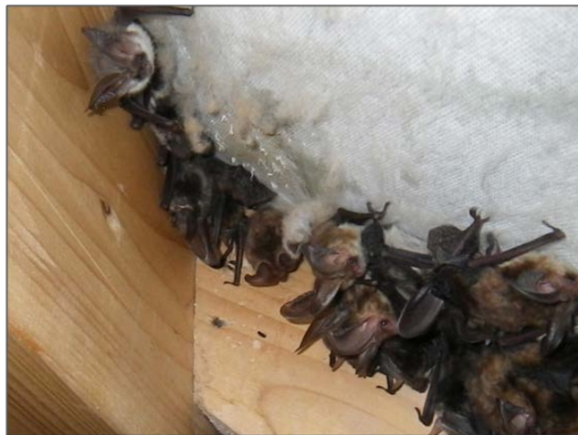
Fig.3. Picture of 'fluffing' on BRM six months after being fitted in a brown long-eared bat roost (Photo Credit - John Martin, 2012, Cumbria, UK)
