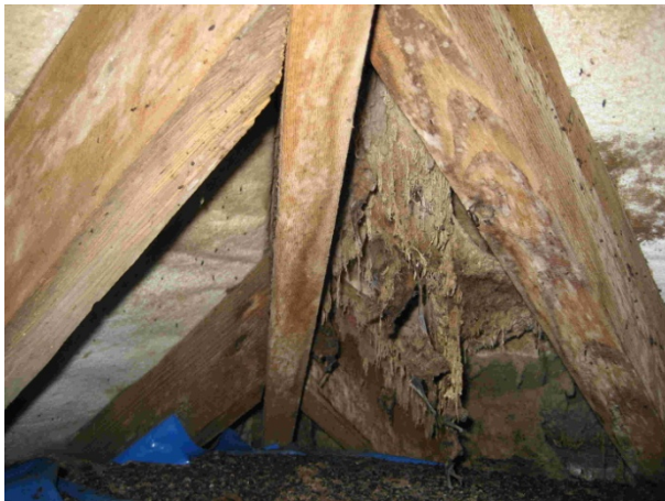
Fig.10. Damaged membrane in which 20 dead bats were found entangled (Photo Credit – Paul Scott, 2007, Dublin, Ireland)
