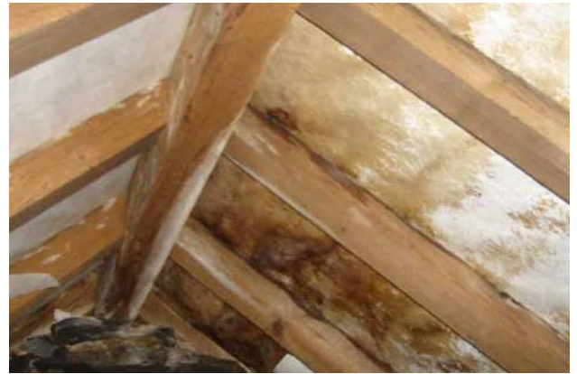
Fig.8. Staining of a BRM through absorption of excrement (Photo Credit - Shirley Martin, 2010, Cumbria UK)
