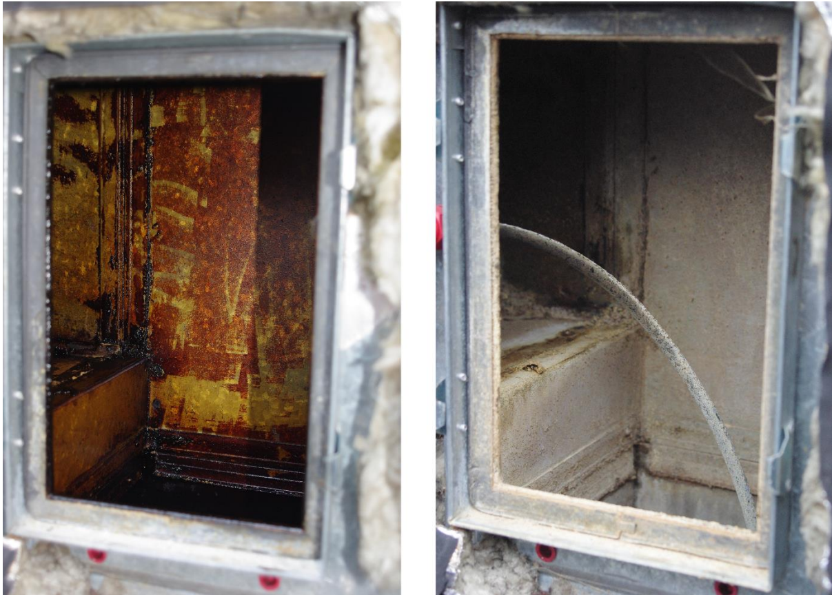
Figure 7: Hatch 1 pre-installation (left) and 2 months post-installation (right)
