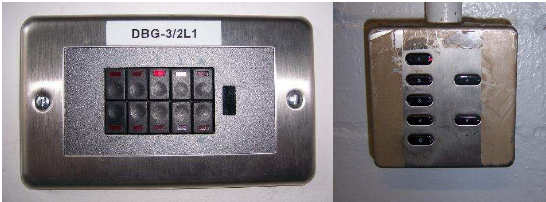
Figure 4. Two specific examples of poor classroom light switches that were explicitly mentioned in relation to participant's difficulty using the controls
