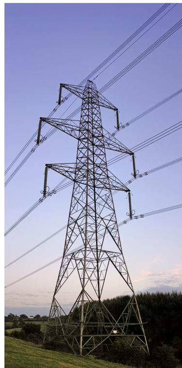
(b) 400 kV L6 D transmission line tower with quad conductor bundles near Aust, Gloucestershire, England<sup>2</sup>
