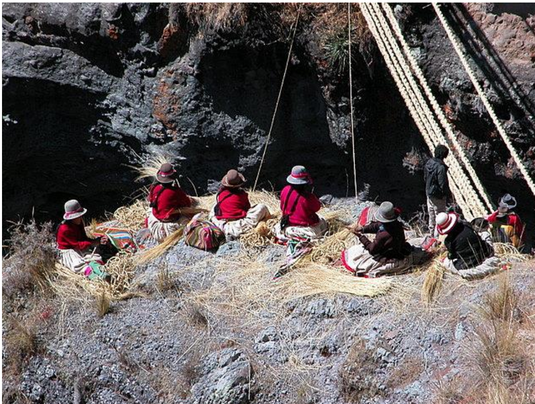
Figure 2 – Women weaving grass rope during the construction of the Keshwa Chaca . (Image courtesy of Ric Finch)
