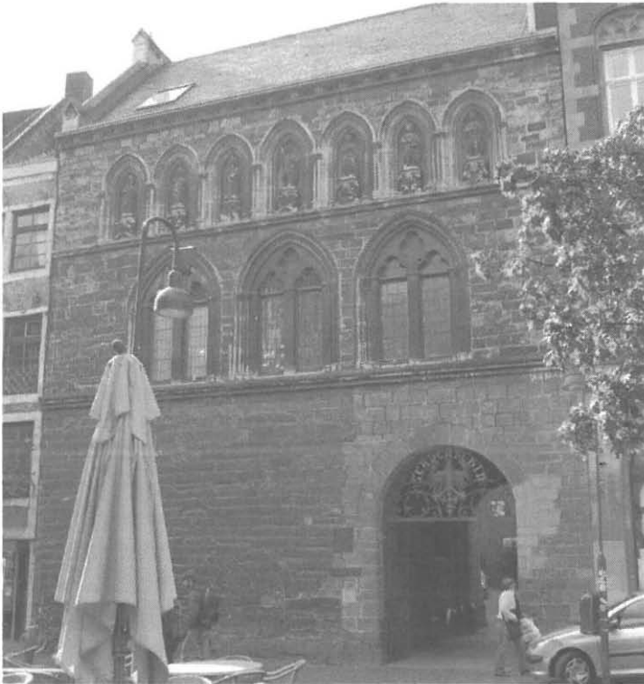
Figure 4: The Aachen Grashaus in the Fischmarkt, built in 1267. Now housing the city-archives, it was the town-hall before the restoration of the ancient Carolingian aula for this purpose in the late fourteenth century. It is heavily restored and the statues of the seven electors are modern replacements of statues known from early drawings.*
