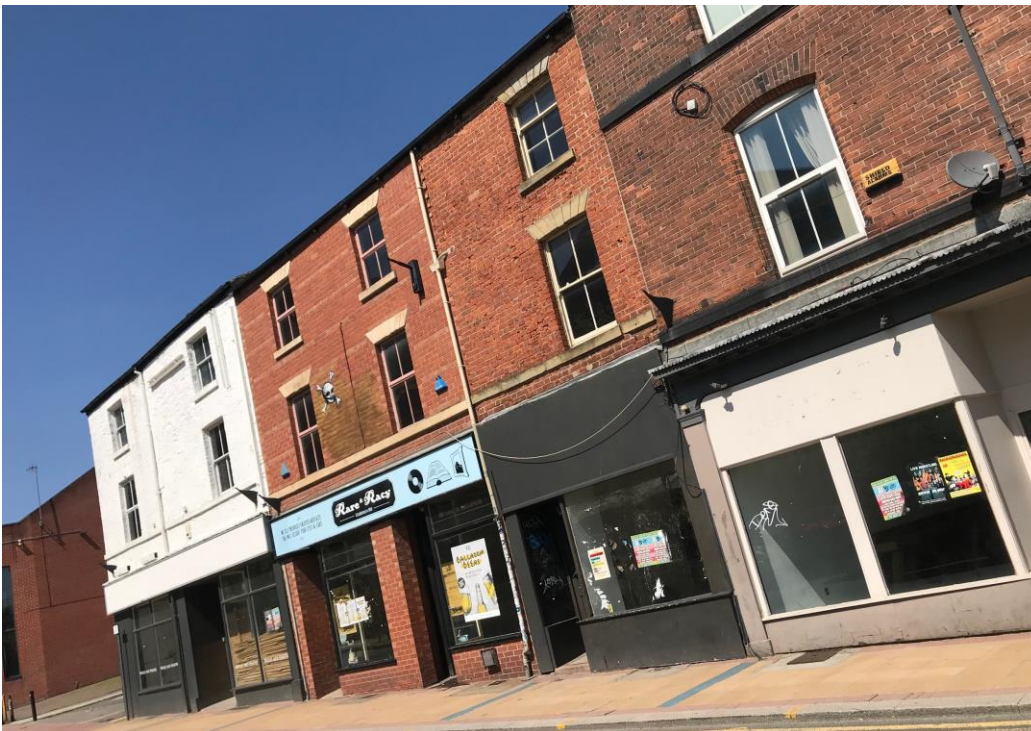
Figure 3: The Existing Front Elevation, including the replacement front wall at 166 Devonshire Street (Source Author, taken May 2018)
