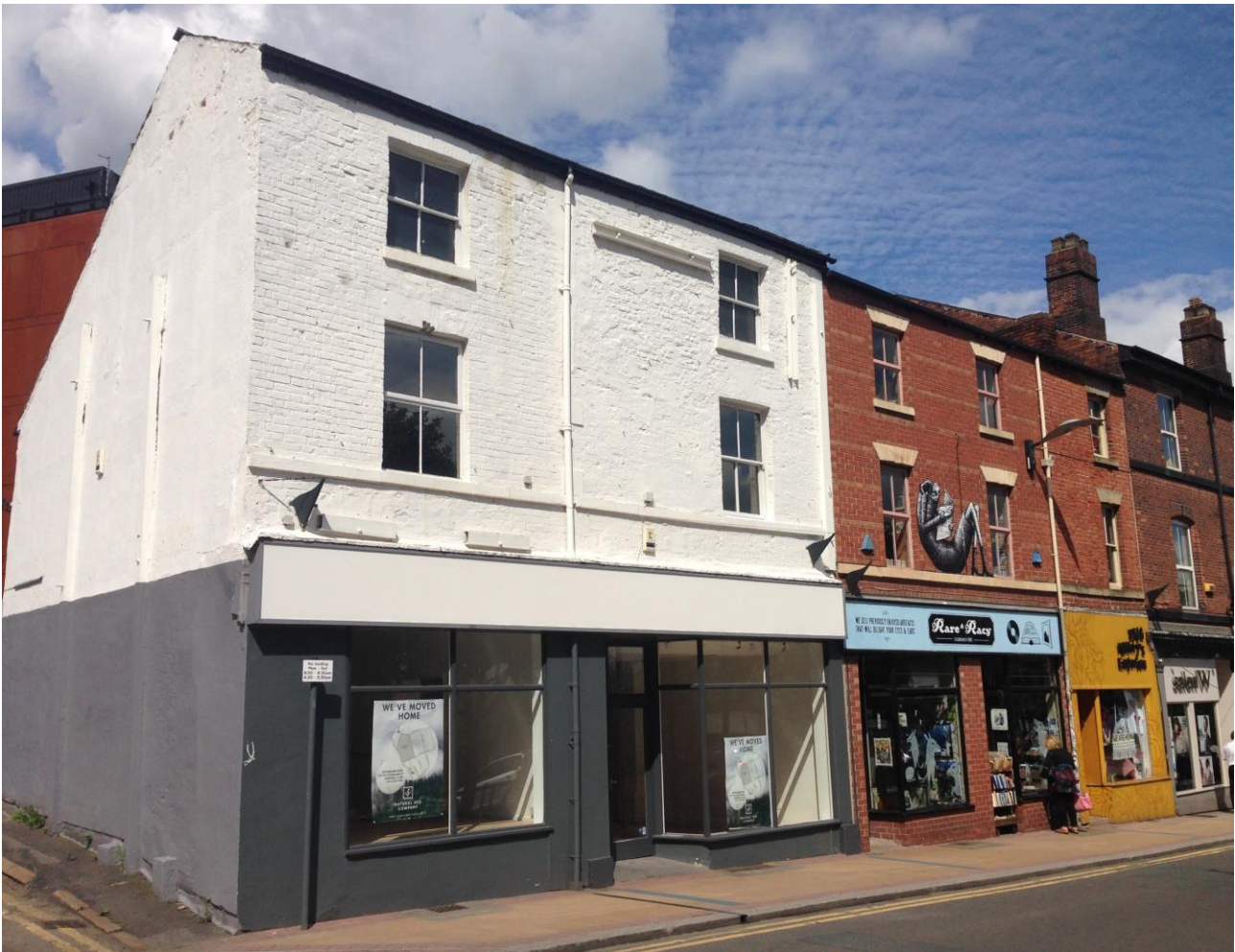
Figure 2: 162-170 Devonshire Street (Source Author, taken June 2016)
